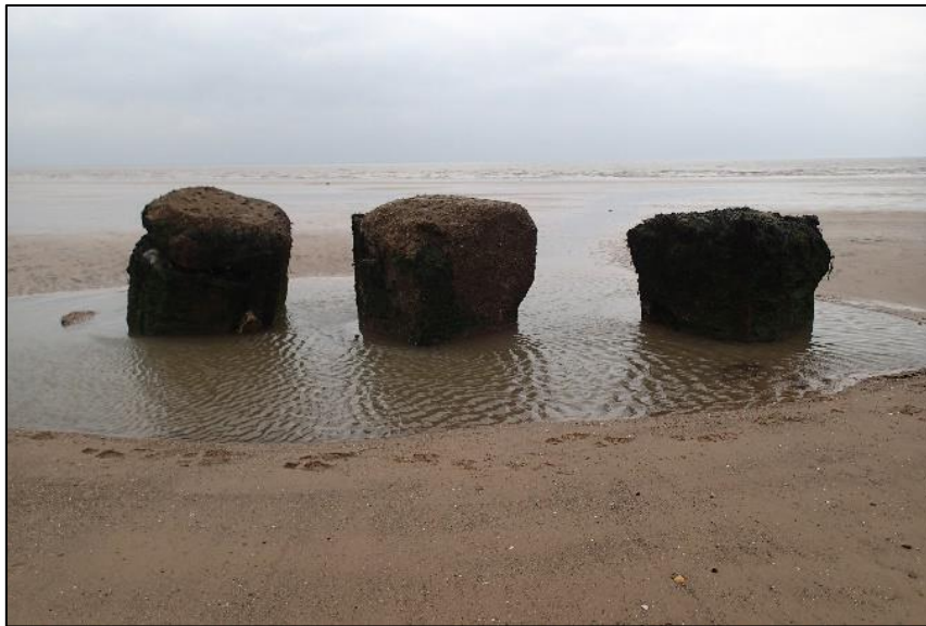
Figure 40: Example of scour around WWII tank traps (IECS 2019).
